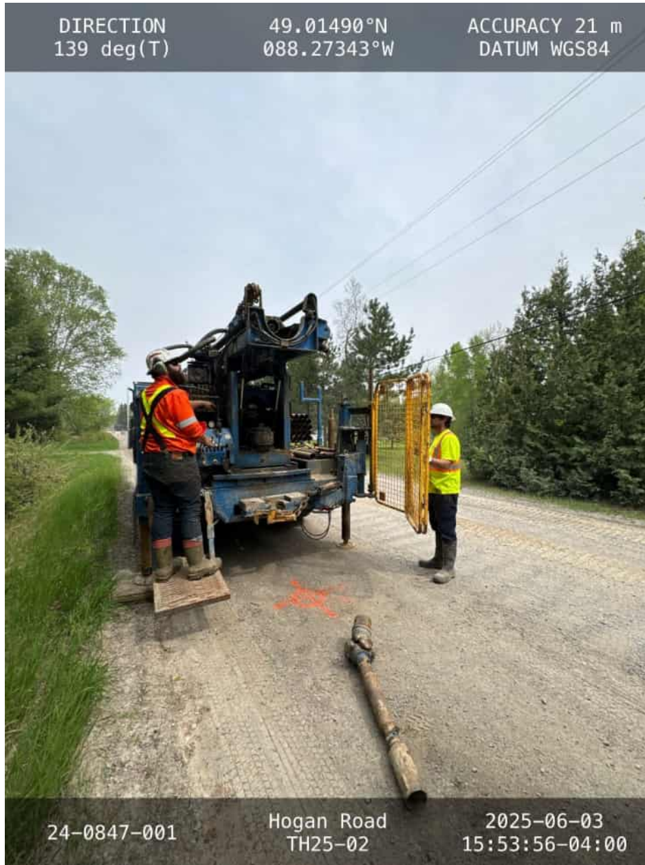
Photo 2: Drill Rig Setup at TH25-02 Located Along Hogan Road, Looking East
