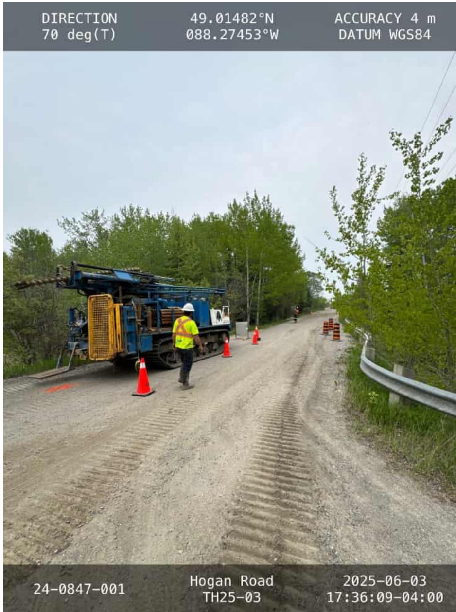
Photo 3: Drill Rig Setup at TH25-03 Located Along Hogan Road, Looking East
